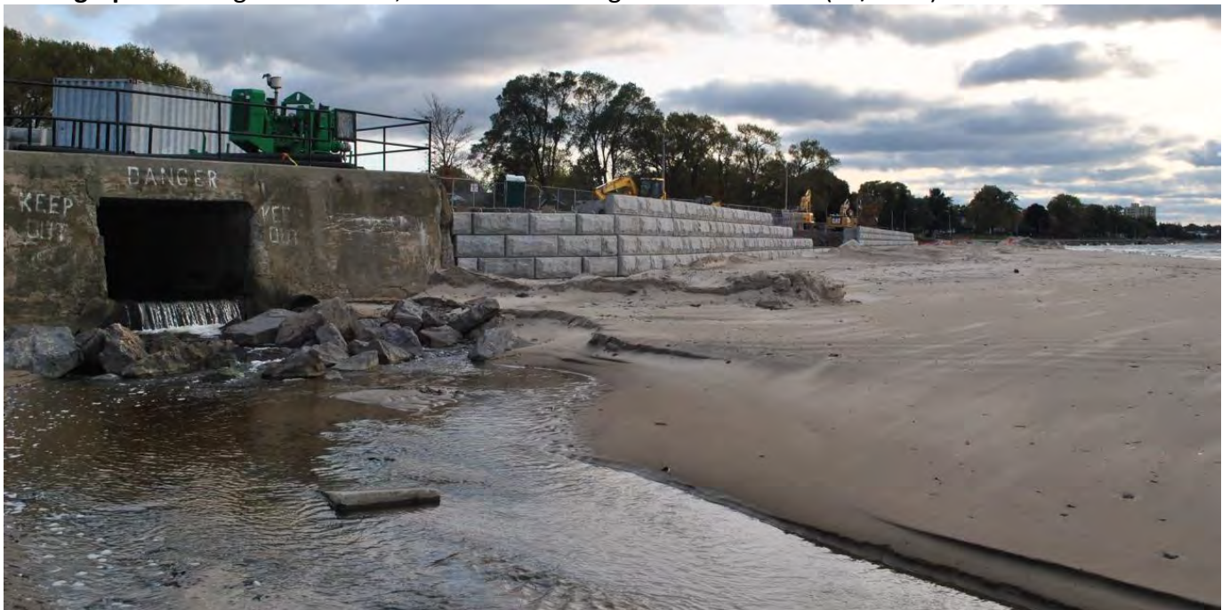
Photograph 25. Wright Park West, new seawall being set and secured. (10/2014).
