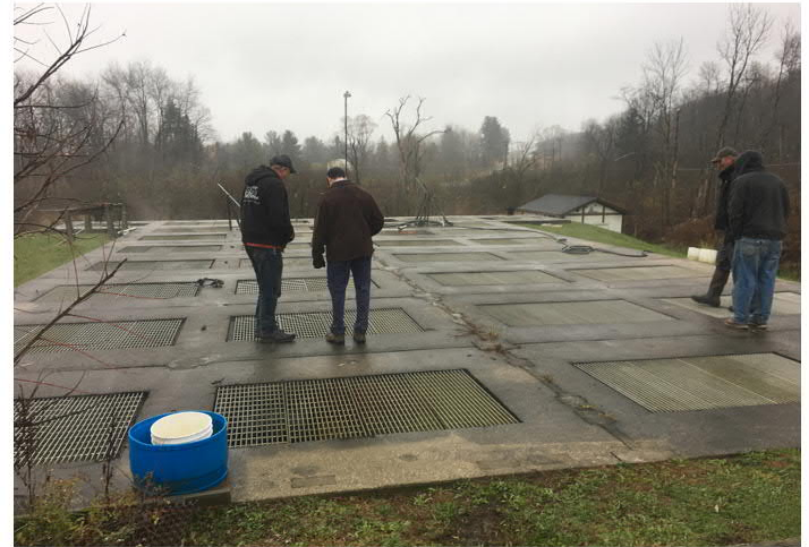
Concrete Aeration, Clarifier, and Settling Tankage
