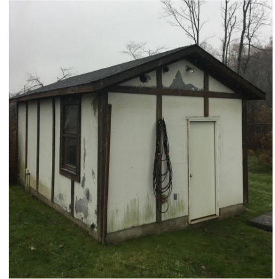
Chlorination and Effluent Pump Station Building
