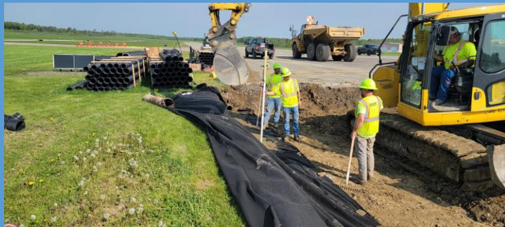
(TOP) MILLED SURFACE AT TAXIWAY B (BOTTOM) UNDERDRAIN INSTALLATION
