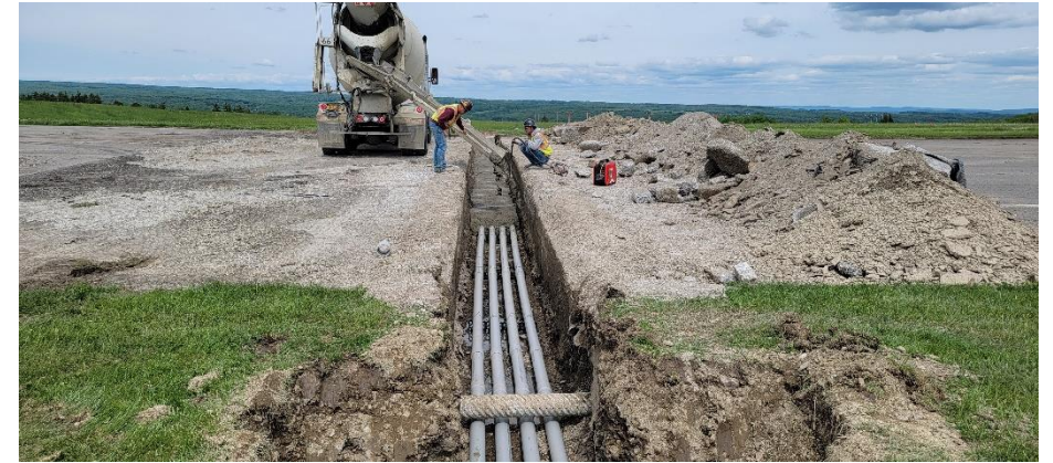
Duct bank installation (Work Area B, across Taxiway D4)
