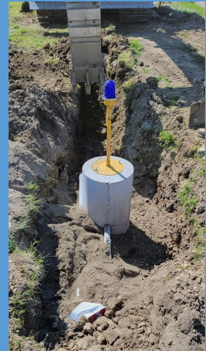
TAXIWAY EDGE LIGHT INSTALLATION AT TAXIWAY A4
