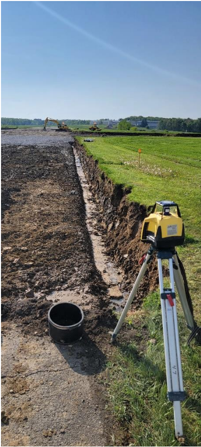
Installation of underdrain (Work Area C)
