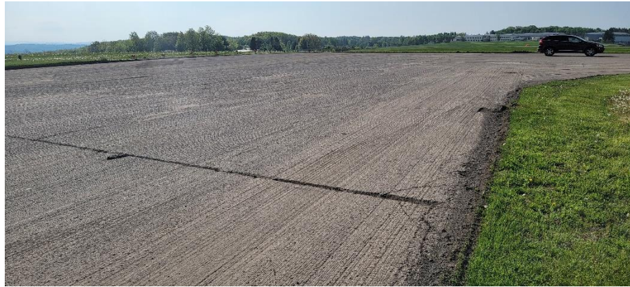
Milled surface in Work Area B (Approach end of Runway 25)
