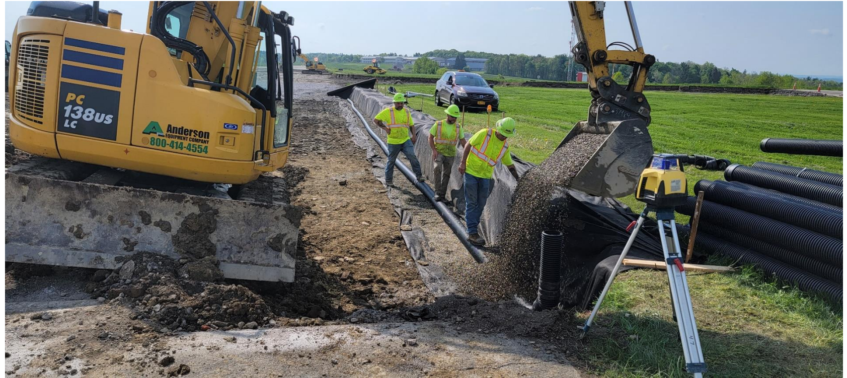
Above: May 23, 2022 status of Runway intersection, underdrain installation
